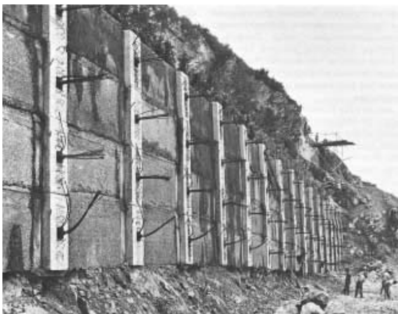
Fig. 31: The wall at Wingreis
