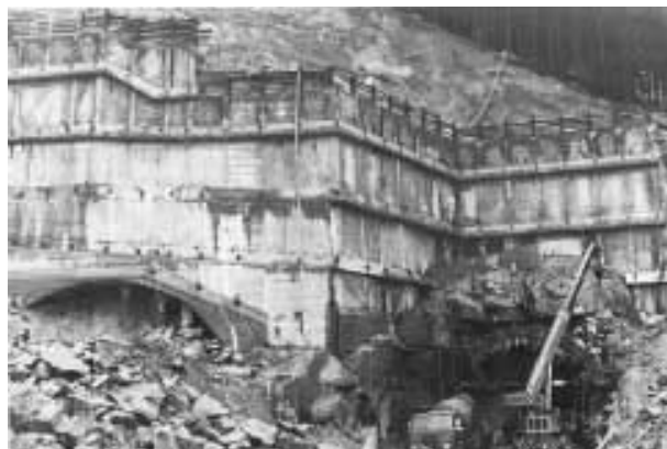
Fig. 34: View of the wall near the tunnel entrance
