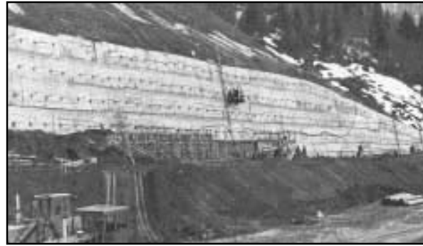
Fig. 26: General view of wall during construction
