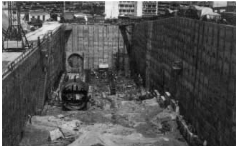
Fig. 44: View of the excavation
