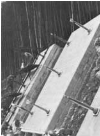
Fig. 24: View of divided retaining wall
