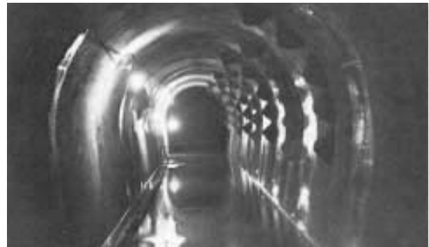
Fig. 17: Drainage tunnel with anchorage blocks
