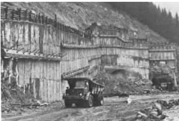
Fig. 33: View of the anchored pile wall
