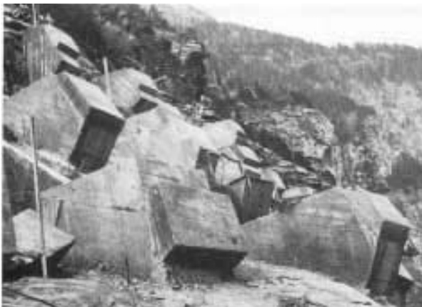
Fig. 6: Anchorage blocks of 1400 kN-anchors
