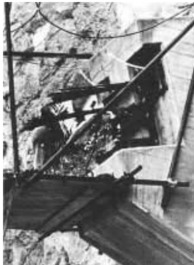
Fig. 73 Anchor work on an upper foundation
