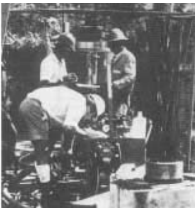
Fig. 86: Stressing operation
