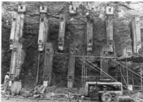
Fig. 27: Anchored concrete tie-beams
