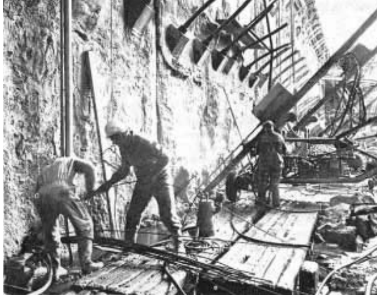
Fig. 48: Execution of the anchor works
