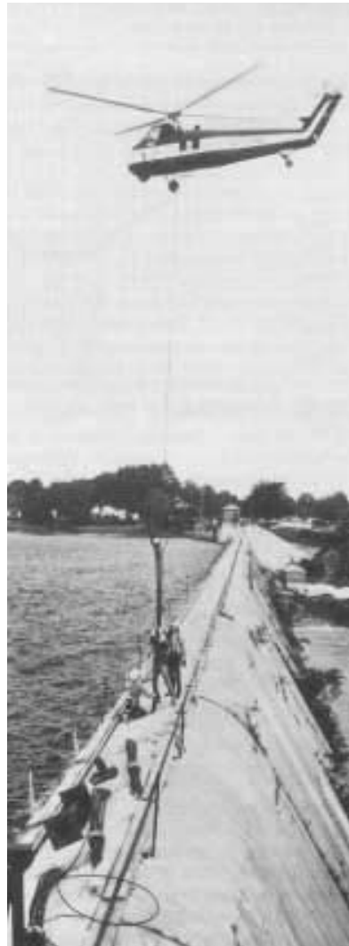
Fig. 83: Positioning of the anchors
