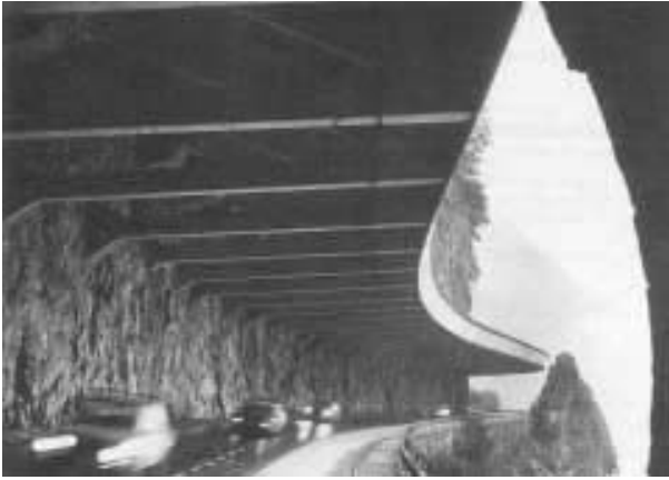
Fig. 71: Partial view of the finished rock fall gallery
