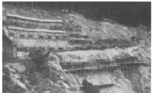
Fig. 13: View of the site at a later stage
