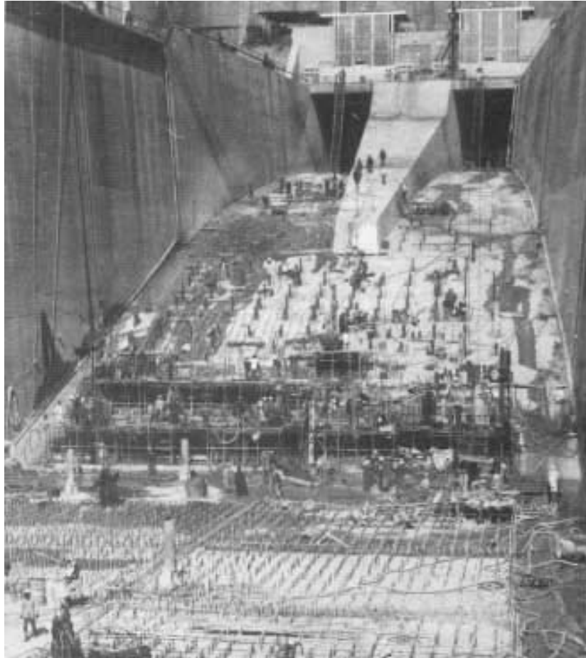
Fig. 57: The stilling basin during anchor work
