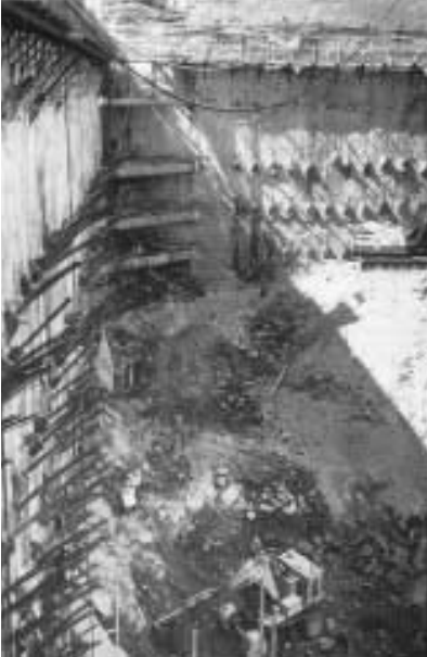
Fig. 47: View of the excavation
