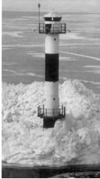
Fig. 77: The lighthouse at Kullagrund
