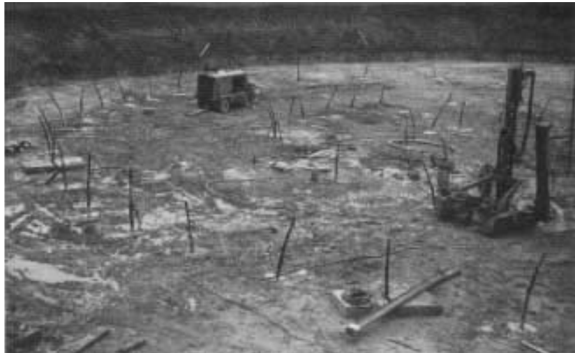
Fig. 52. View of the site with installer anchors
