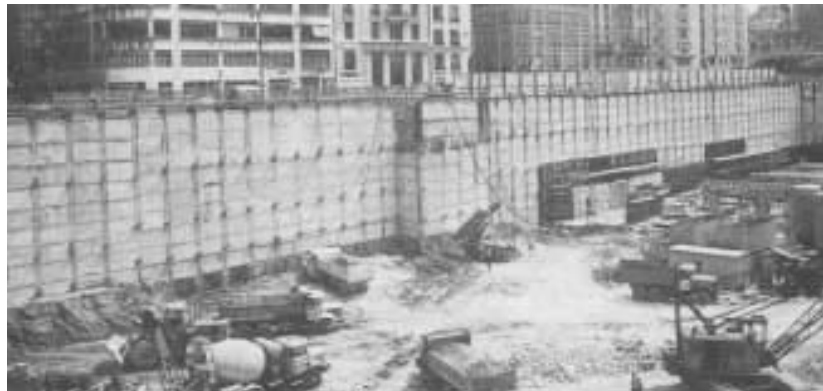
Fig. 39: View of the wall
