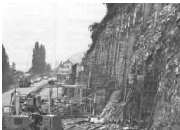
Fig. 29: Construction of staggered wall
