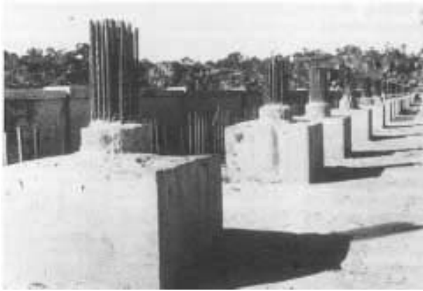
Fig. 87: View of anchor tops
