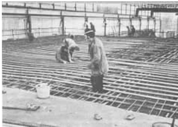
Placing of transverse cables
