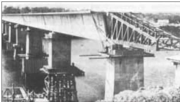
Fig. 2: Bridge over the Rio Caroni, Venezuela
