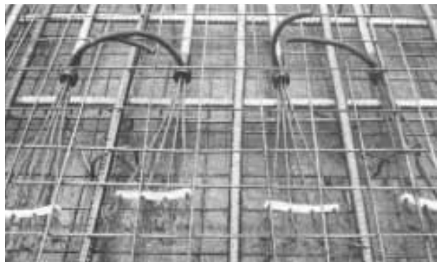
Fixed anchorage type HI of transverse cables
