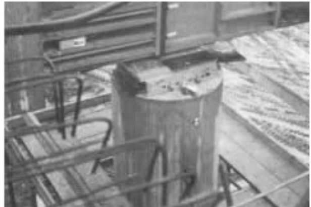
Bearing with sliding plates
