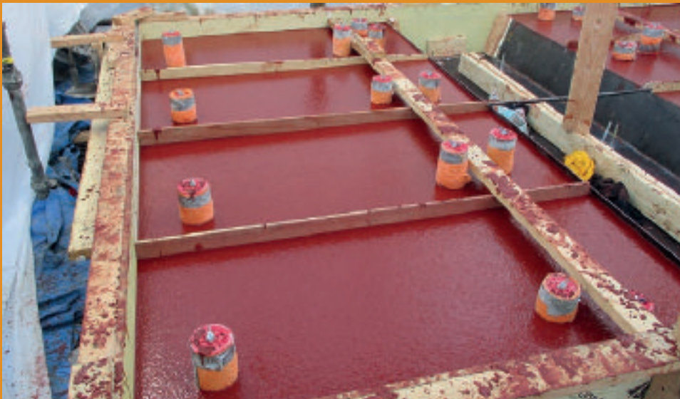
Grout installation with expansion joints and anchor bolt sleeves.
