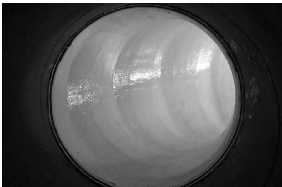
Figure 9. Completed CFRP lining
