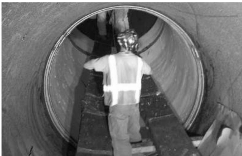
Figure 7. Access planking system to allow for full circumferential access to the work scope
