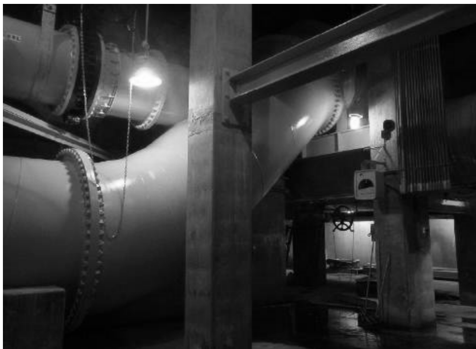
Figure 5. Outside view of vertical bend regions of Nit RAS pipeline repaired internally with CFRP
