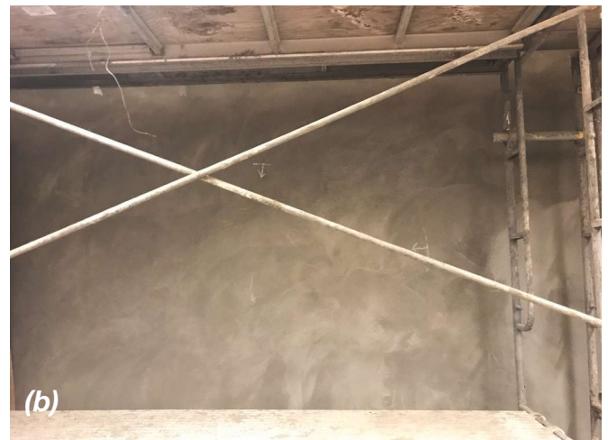
Fig. 7: Wall before (a) and after (b) installation of FRCM final finished layer
