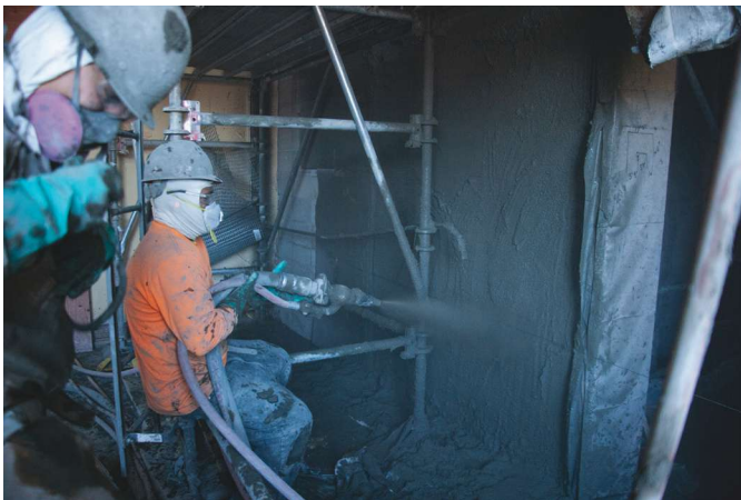
Fig. 5: FRCM application over the prepared surface
