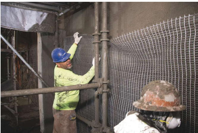
Fig. 6: Laying out and wet-set of unidirectional carbon grid
