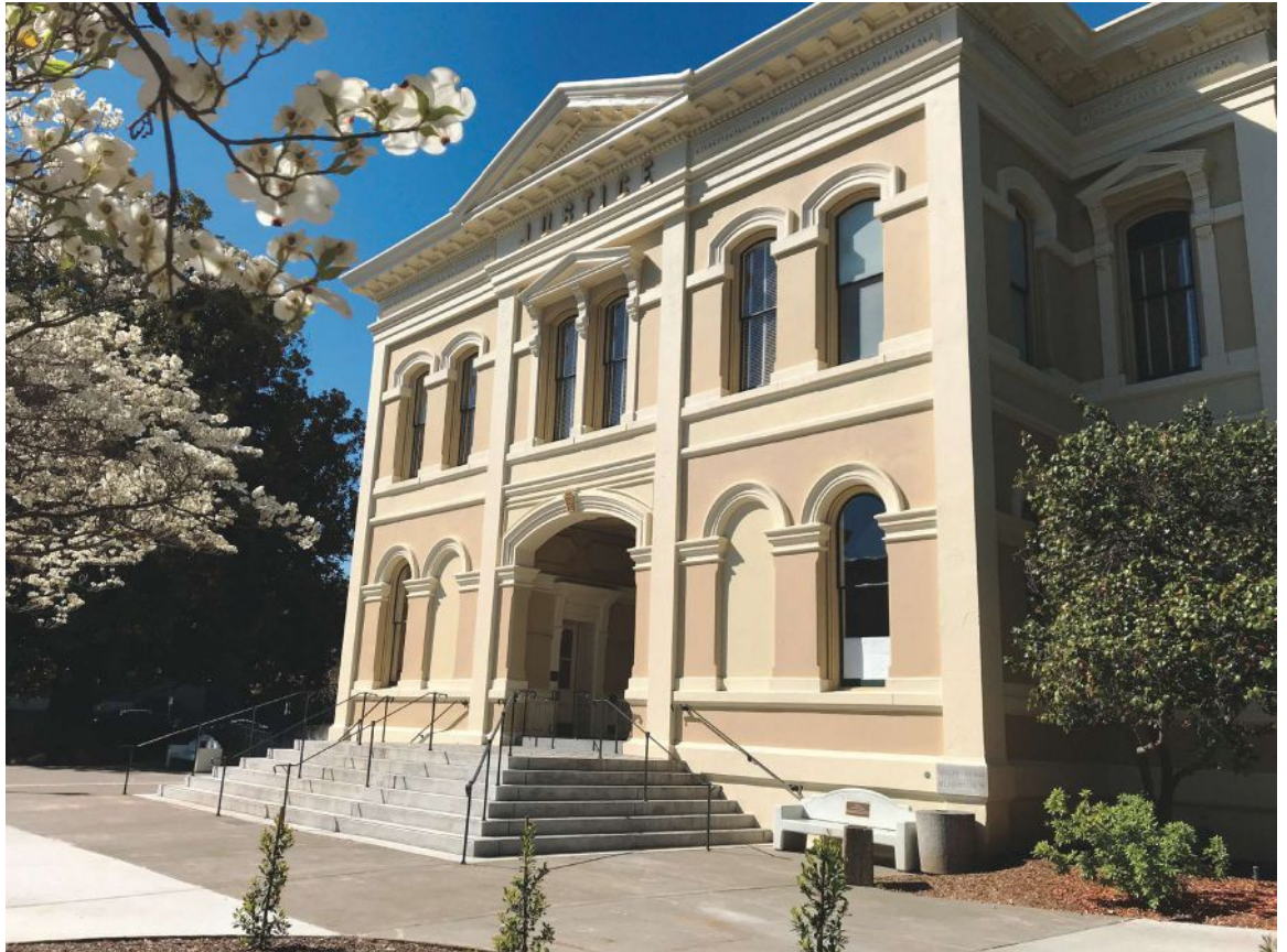
Fig. 1: Napa Valley Courthouse after repairs
