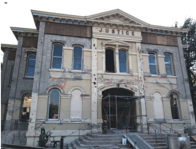
Fig. 7: The Courthouse construction near completion
