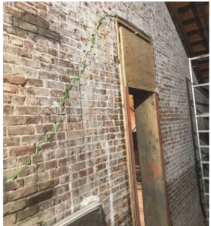
Fig. 3: Traditional masonry repair strategies, including grout injection and masonry ties, stabilized the structure to receive seismic upgrades
