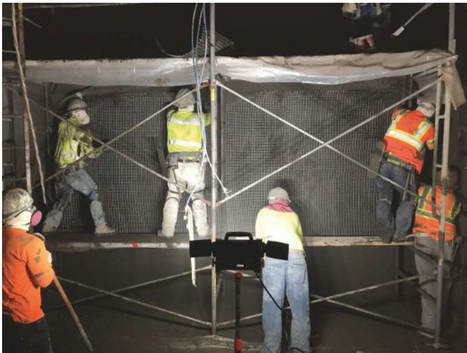
Fig. 5: Reinforcing a wall with the FRCM system
