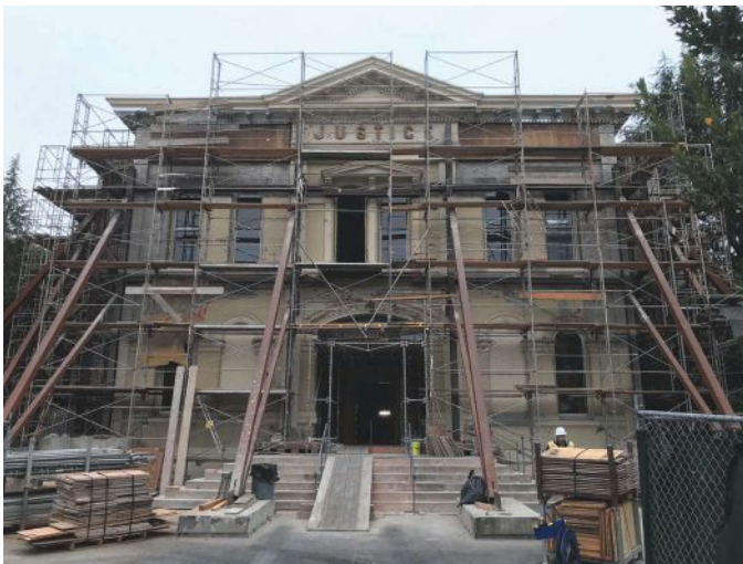
Fig. 6: The Courthouse after removing the sheathing, and prior to exterior plaster and coating work
