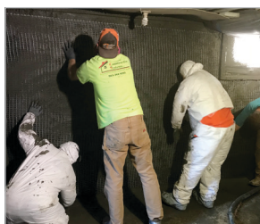
Installers pressing the carbon grid (CSS-UCG) into the first layer of the wet-set cementitious matrix (CSS-CM).
