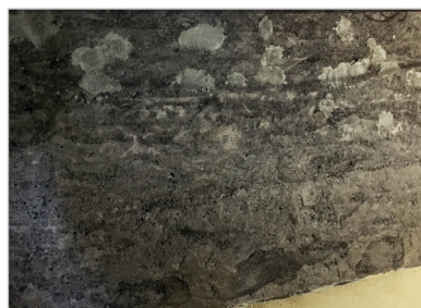
The unreinforced concrete walls before FRCM treatment.
